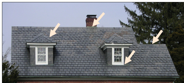
The arrows indicate areas where flashing is typically located.
