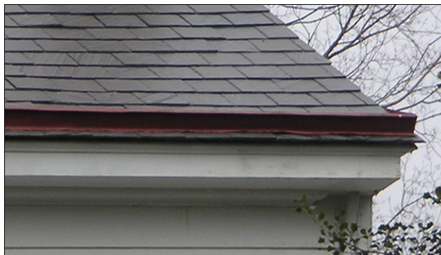
Pole gutters, also known as parallel gutters, are built-in gutters located near the roof edge to capture rain water and direct it towards a downspout. They are typically formed of wood, placed vertically to the slope of the roof and wrapped in metal flashing.
