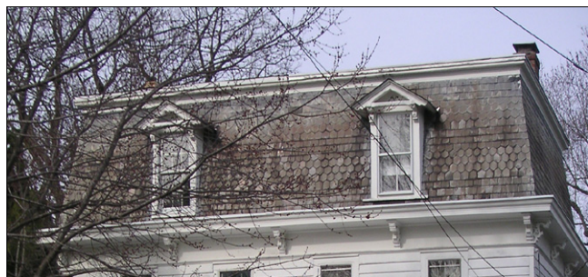
This mansard roof features rectangular and octagonal slates and has a flat upper roof that is not visible from the ground.
