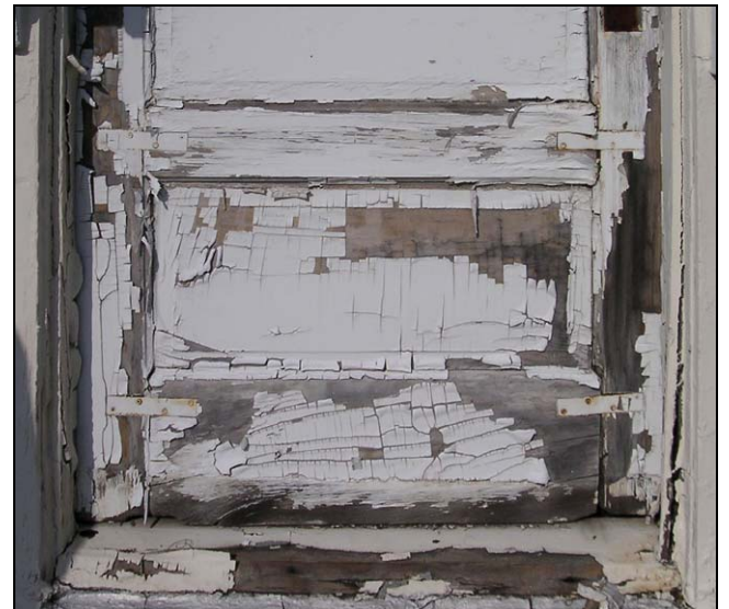
The paint on this door has alligatoring, and severe cracking is visible. Removal of paint down to bare wood and proper door repair are recommended before repainting
