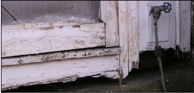
The wood base is in contact with the concrete foundation. Regular wood dampness can eventually lead to rot and deterioration.
